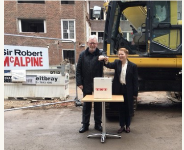
Ex Yorkshire House Construction Manager Commences Demolition 2017
